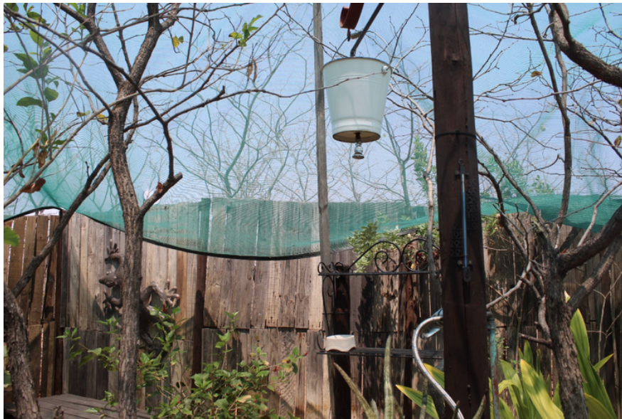
Figure 6: Ablution block at The Plot, in the outskirts of Letlhakane
